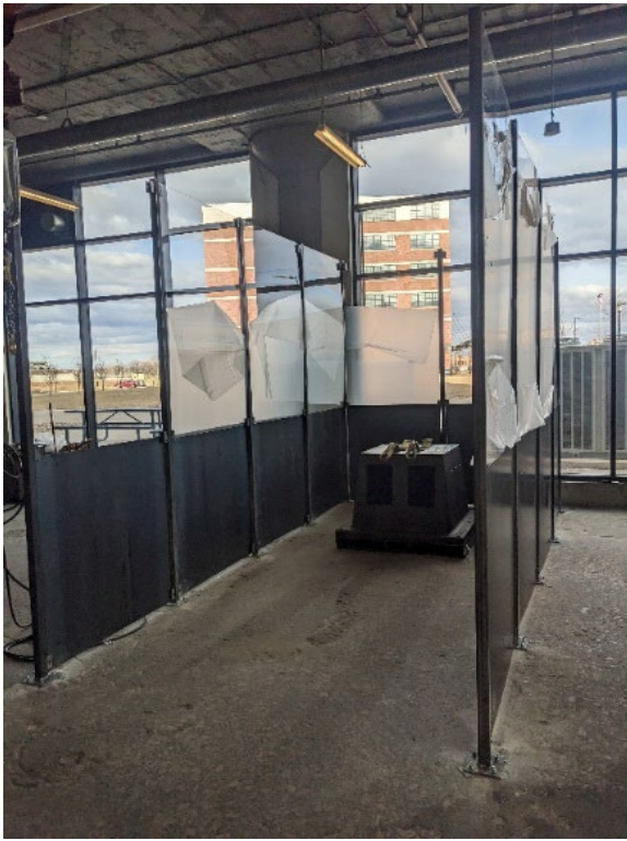
Figure 2. Construction of the cell walls and placement of the working pedestal.
