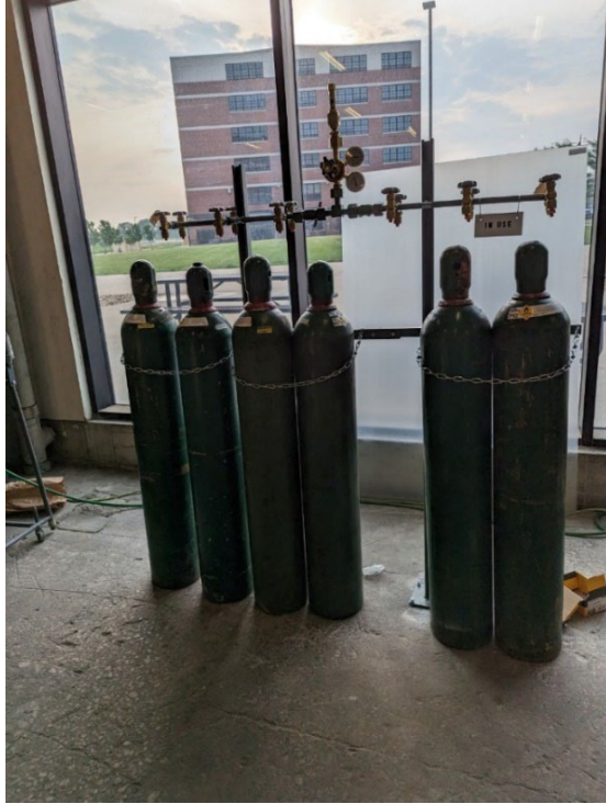
Figure 8. Oxygen delivery manifold leading into full gas manifold.
